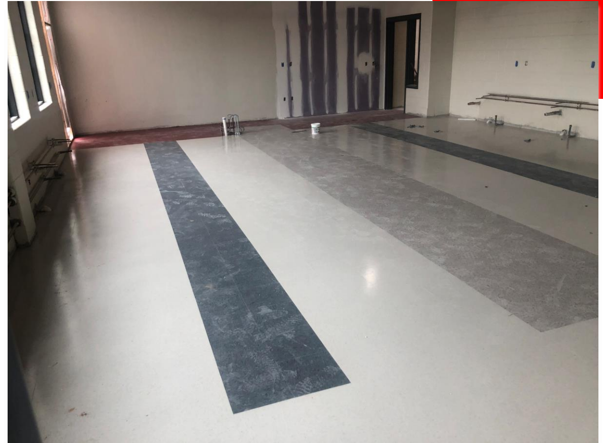
VCT Installed in 4 th Floor Classrooms of New Addition
